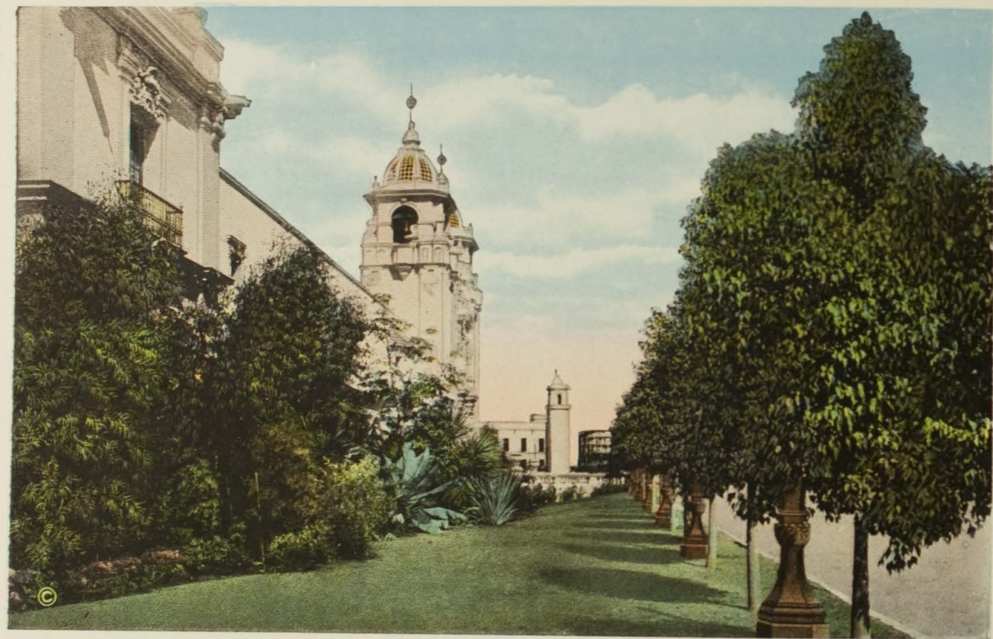
Vista along East Side of Varied Industries Building, looking North.
