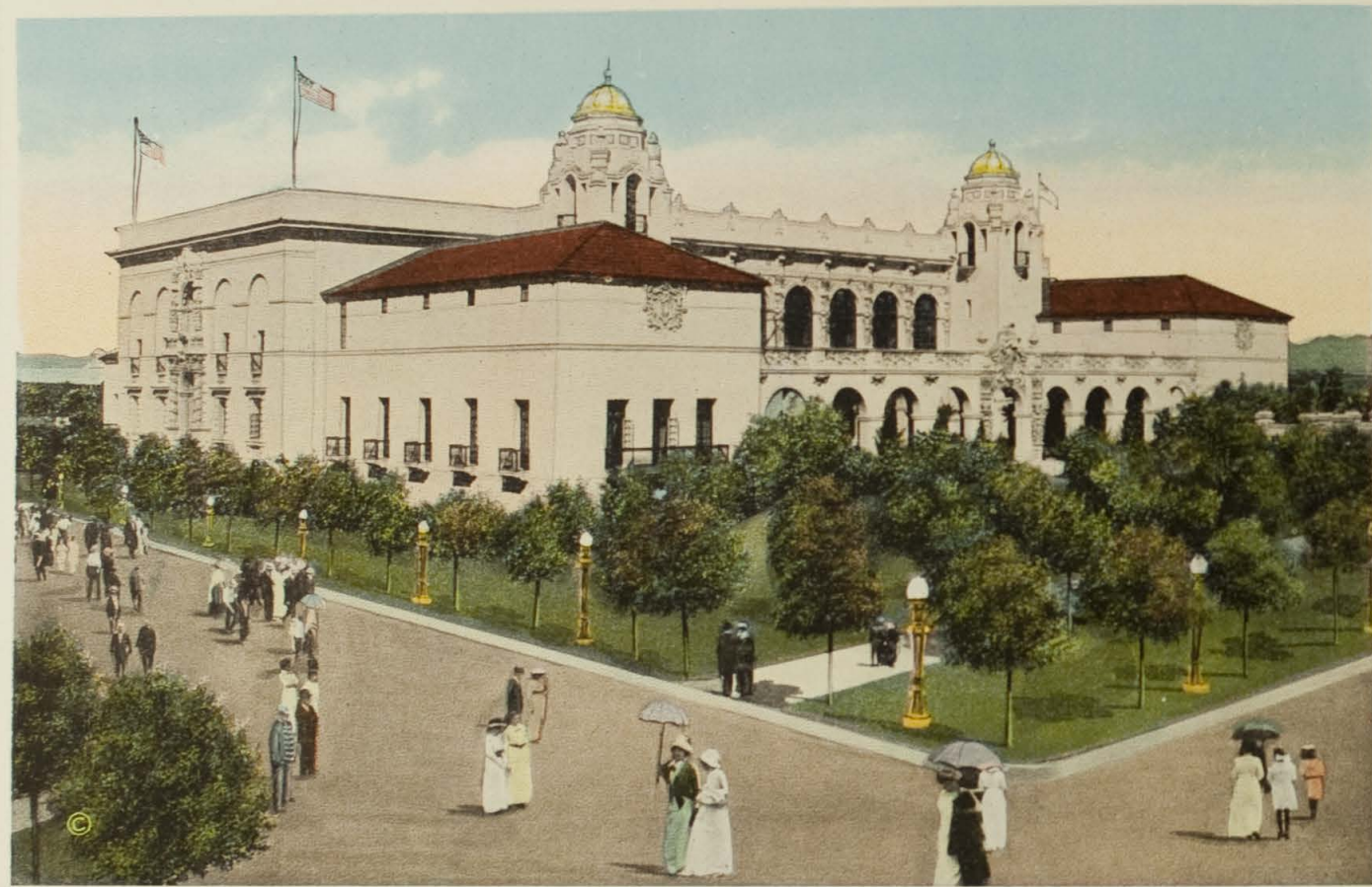
Building erected by Seven Southern Counties of California.
