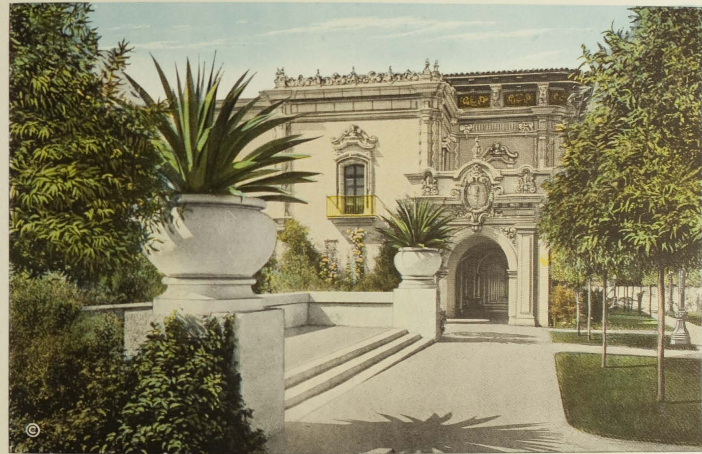
East Entrance to Commerce and Industries Building Colonnade
